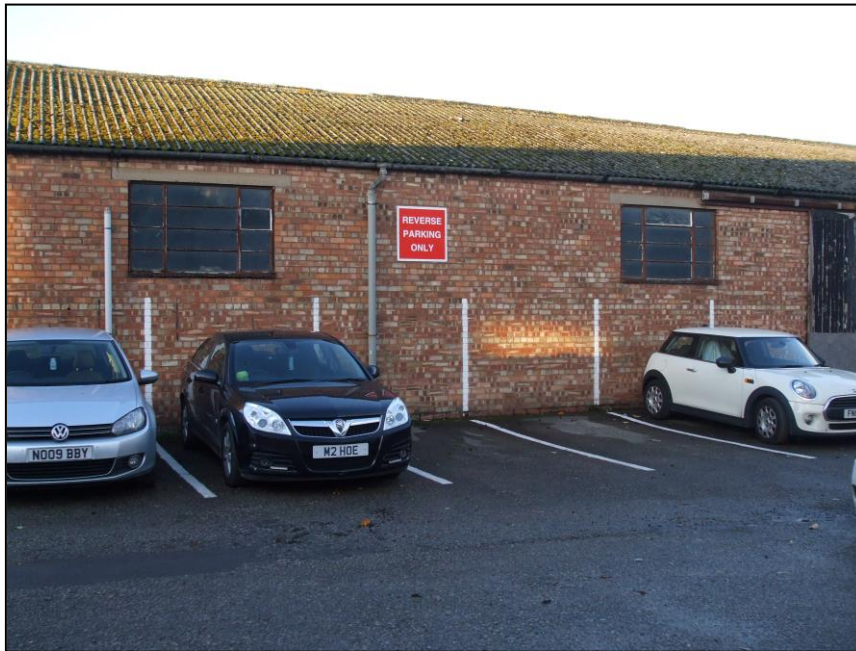
Photograph 1 – Existing building to be demolished
